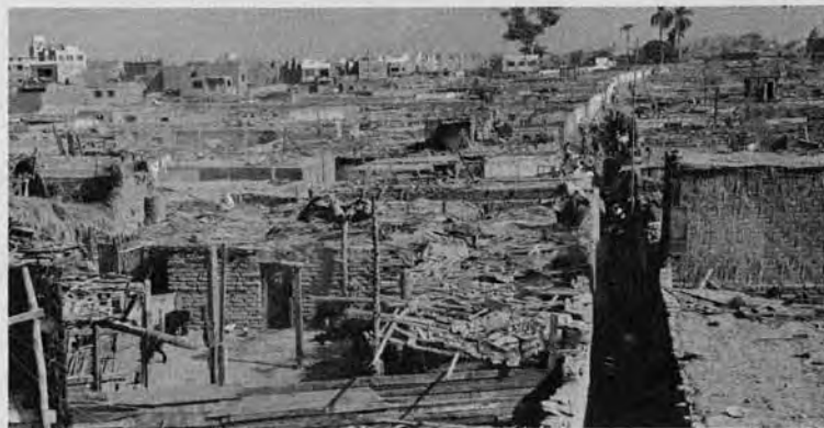
PLATE 9. A barriada , or squatter settlement of the poorer sort, in Lima, Peru. Note the middle-class neighborhood in the background—which provides many of the settlement's inhabitants with job market. JOHN F. C. TURNER
